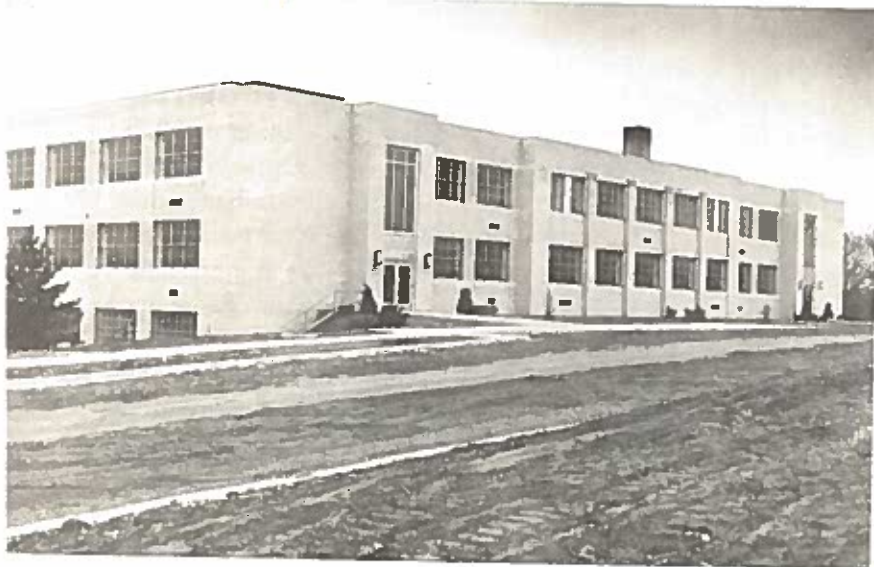
View of the "New West Lafayette High School" completed in 1939, at a cost of $225,000, of which the WPA paid 45% and the city and school corporation paid 55%. It was constructed of cream brick and glass and faced Leslie Avenue. Photo, ca. 1940, Tippecanoe County Historical Museum.
