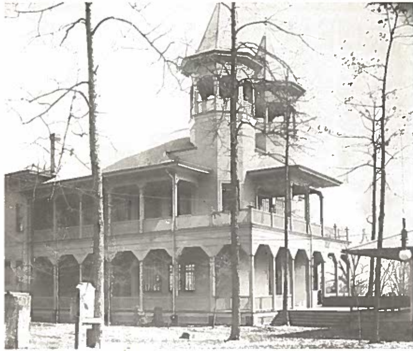
Tecumseh Trail Park Pavilion, across from Soldiers' Home, State Road 43 North. Dedicated June 3, 1897, burned August 12, 1919. Photo, 1897, David Chambers Collection.
